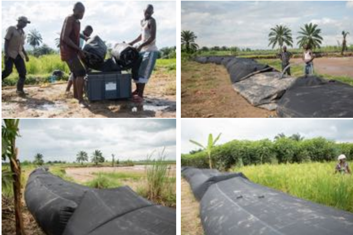
Figure 3: Deployment of the mobile flood barrier the pilot project in Burundi during in 2022
